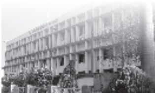
Corporate Office & Works (J-7, Hingna, MIDC)
